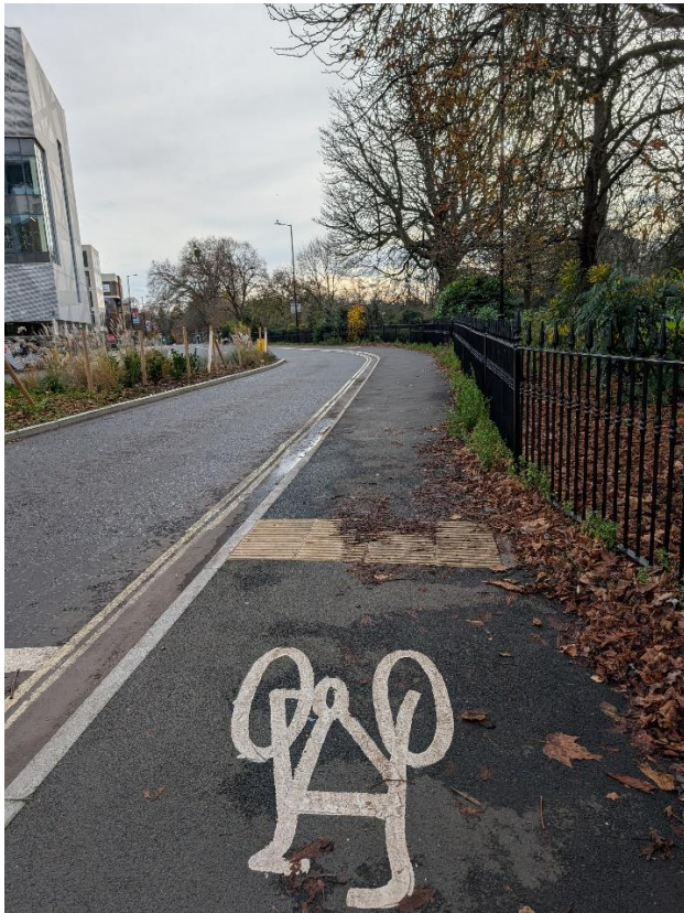
Photo 6 – a new cycle path on East Park Terrace
